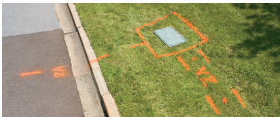
Example of structure, standard marks, corridor
